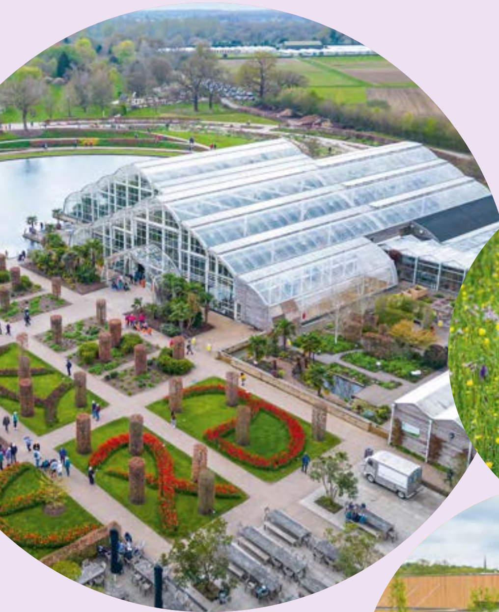
Aerial view of The Glasshouse at RHS Garden Wisley
